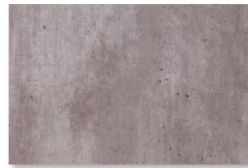
2204-K00 S Cracked Cement
