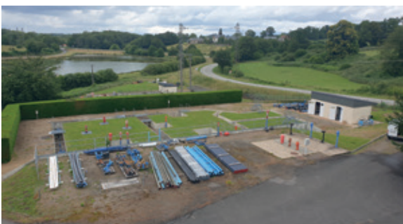
OiEau educational units for "Drinking water supply systems" and "Sewage systems". ©OiEau
