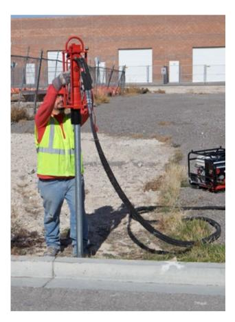
Driving down posts or rods for fences, road signs, crash barriers, tent anchors, or other purposes calls for a tough machine with plenty of power.
