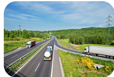
6. Violating Right of Way
