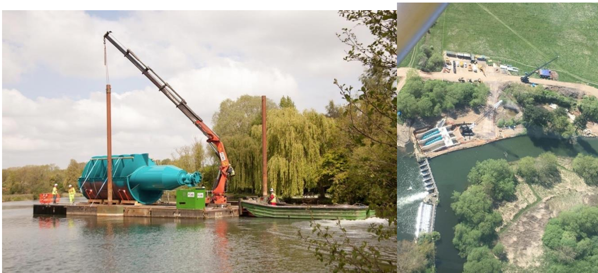
Figure 1: One of the Archimedes screws being transported to the Sandford Hydro site via barge along the Thames (left) and an aerial view of the site, including the weir (right) (Source: Low Carbon Hub)
