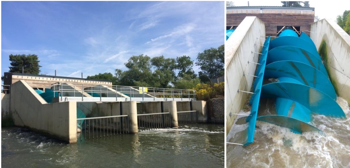
Figure 2: Tailgate view of the Sandford Hydro Archimedes screw (left) and a close-up view of one screw at the site (right)
