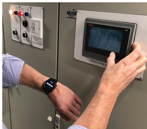
Manual HVAC control in Sackler Library as part of the OBM MVS trial.
