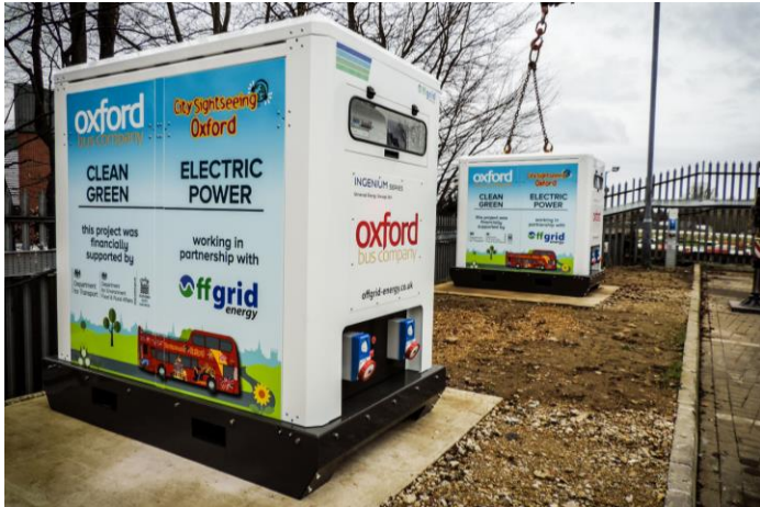
Oxford Bus Co. Batteries (Storage)
