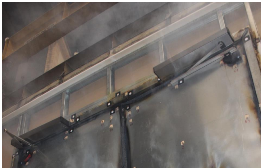
Photo 4: Detail view after test end
