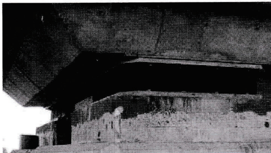
Fig. 1. Laminated rubber bearing.
