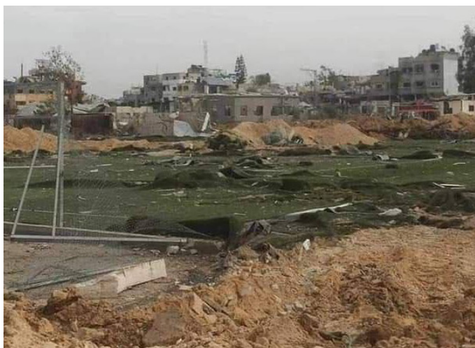
Road and school destroyed in Beit Hanoun
