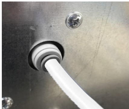
Water Connection at Boiler
