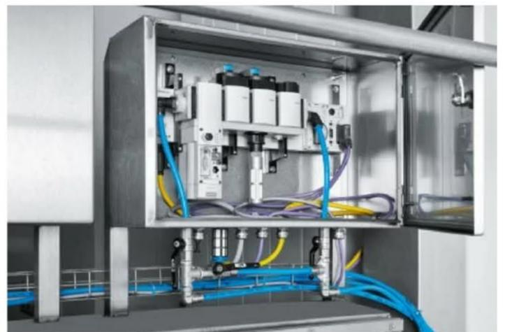
The first generation of the energy efficiency module MSE6-E2M is currently in continuous operation at Unilever. The market-ready module is around 50 percent more compact.
