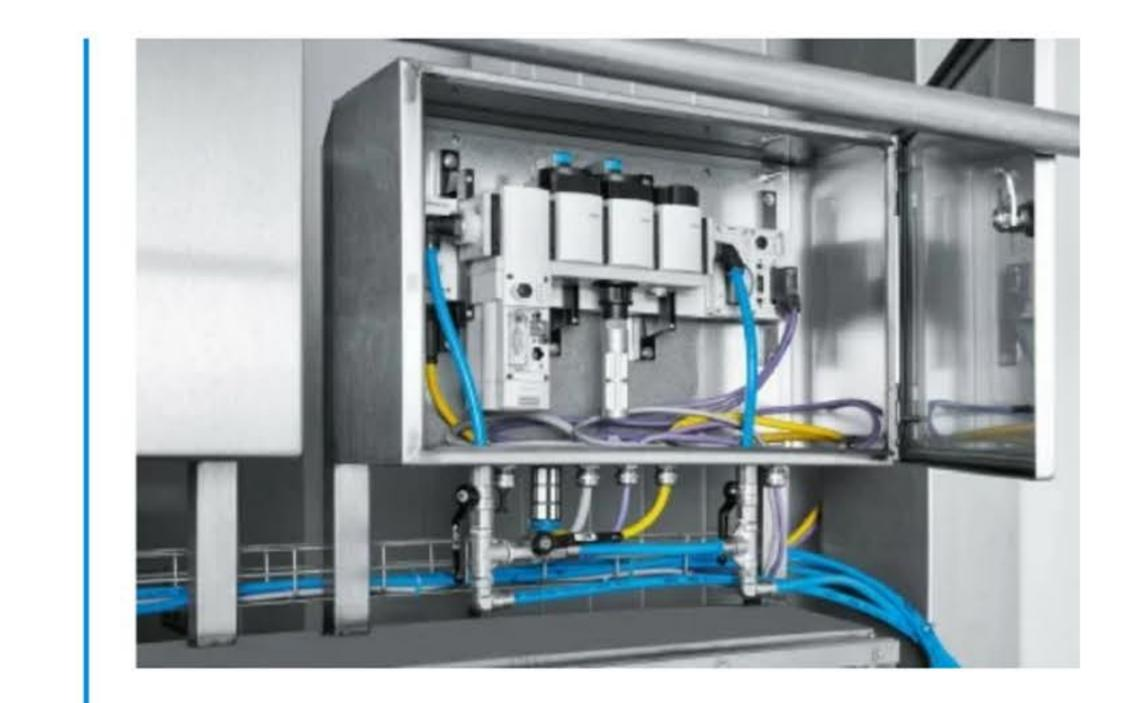
The MSE6-E2M prototype underwent field testing in the Magnum line at Unilever, providing an ideal setting for evaluation. Close collaboration with Festo developers and its pilot use in the Heppenheim plant unveiled crucial operational requirements. As a result, the final version of the energy efficiency module, MSE6-E2M, was refined to better suit daily operations.
