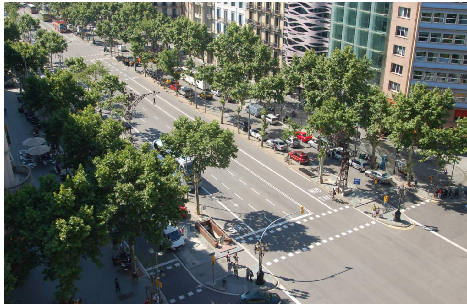
Multimodal boulevard with bus lanes, enhanced bus stops, continuous tree canopies, protected median refuges
