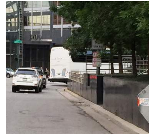
Missing sidewalk segment
