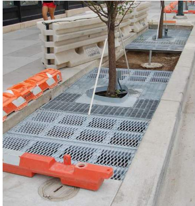
14th Street soil trench with enlarged paving grate (construction)
