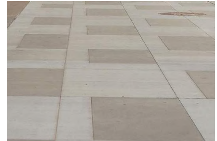
Sawed and sandblasted concrete paving
