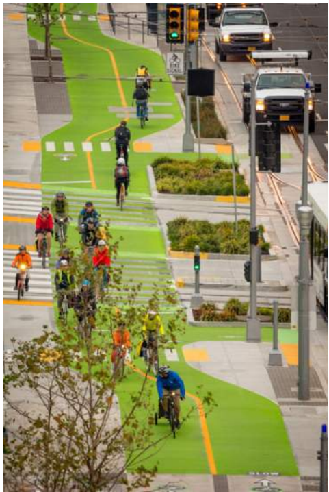
Major protected bike facility integrated with pedestrians, transit and traffic
