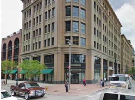
Denver example of appropriate street level design
