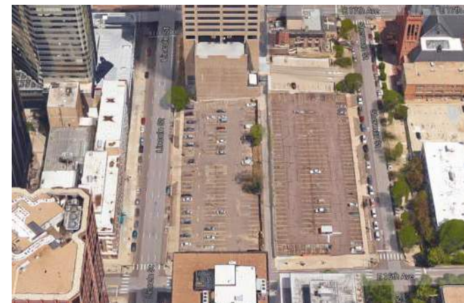
Parking lot at Development Sites 2 and 3
