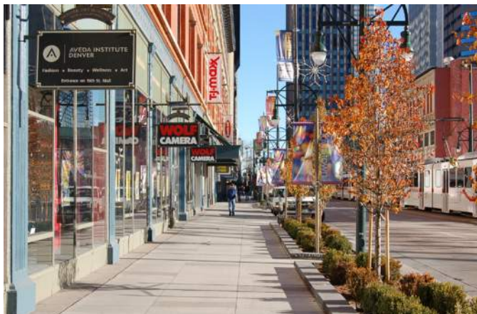
Open tree well - curbed: Denver example uses curbs to redirect contaminated storm runoff
