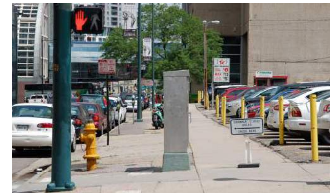
Non-conforming parking lot, clumsy utility location
