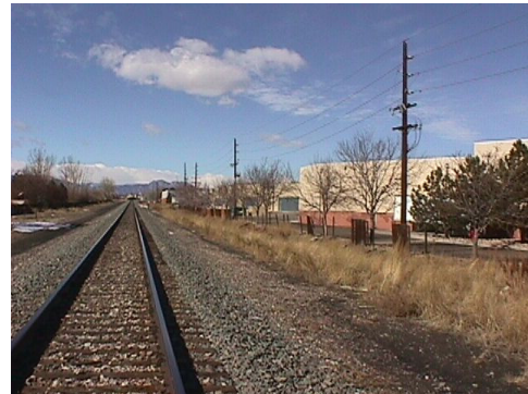
BNSF Railway Company ROW Behind Westminster Mall
