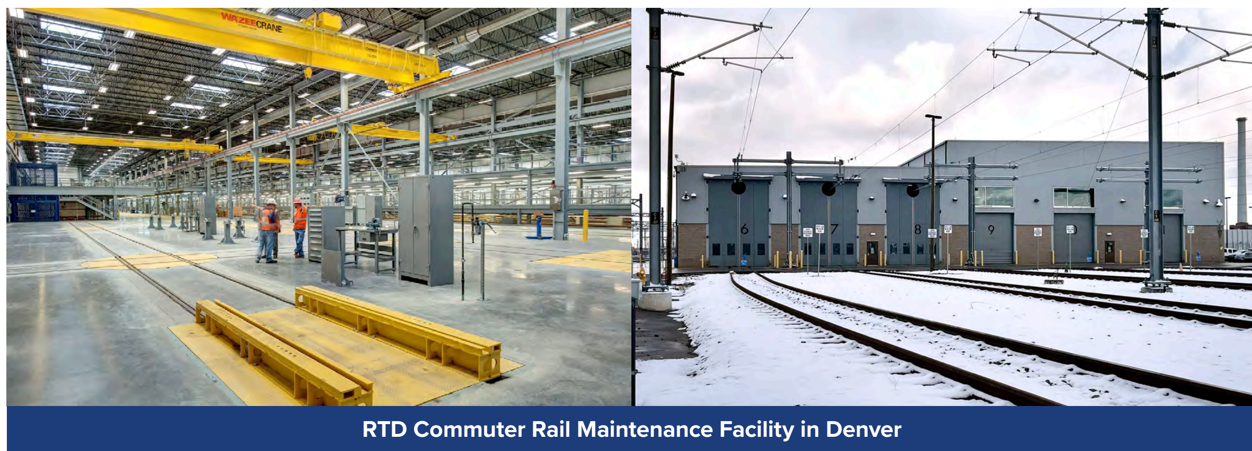
RTD Commuter Rail Maintenance Facility in Denver
