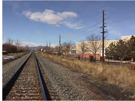
BNSF Railway Company ROW Behind Westminster Mall
