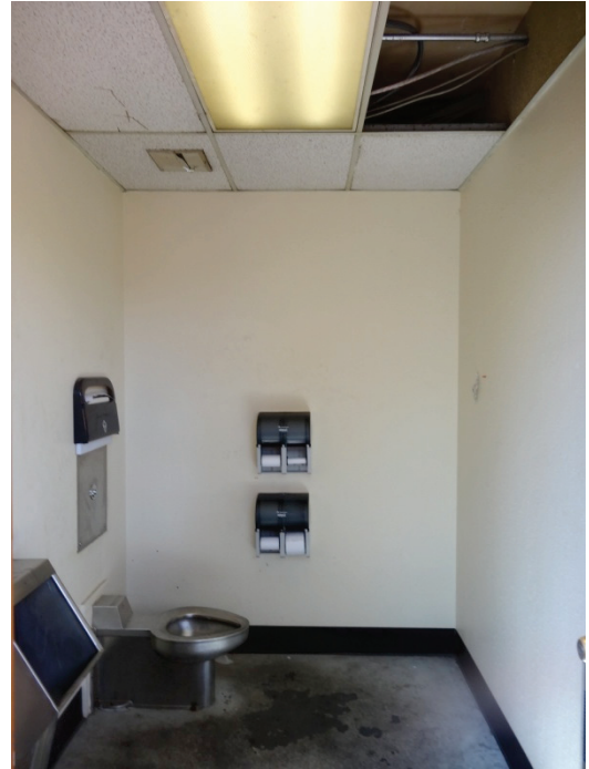
Figure 19. Men's bathroom located at Gate 1 (location a), primarily used by truck drivers. It features stainless steel fixtures, including a toilet with non-operable seat.
