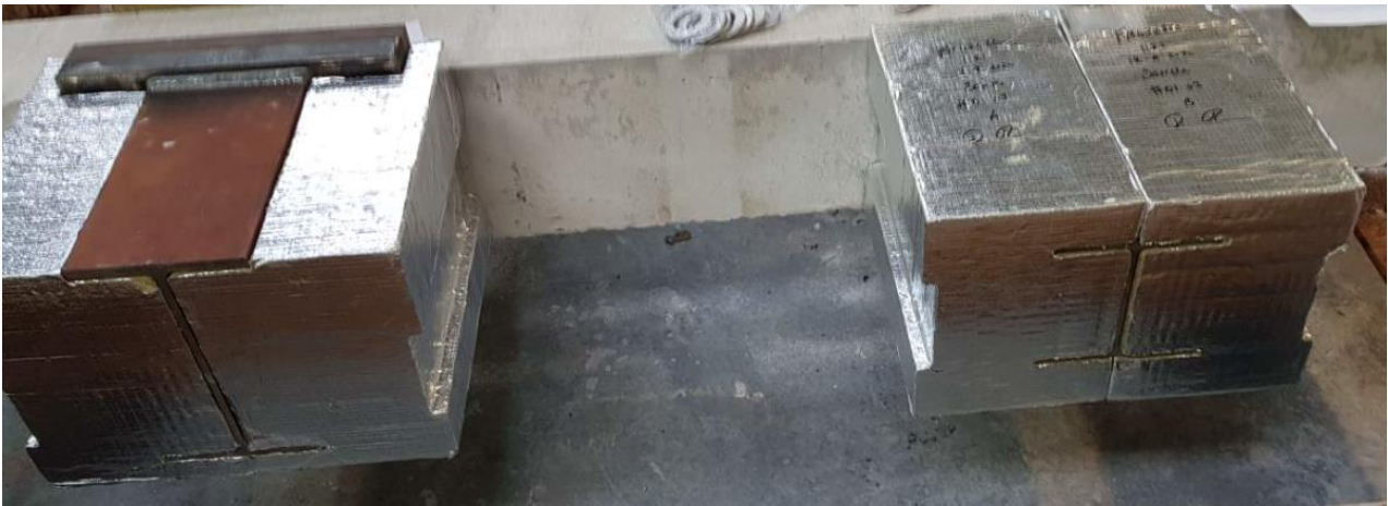
Fig 3 Stubguard® being fitted prior to cavity fire barrier fitting (Foil to front face may be omitted without affecting fire performance)
