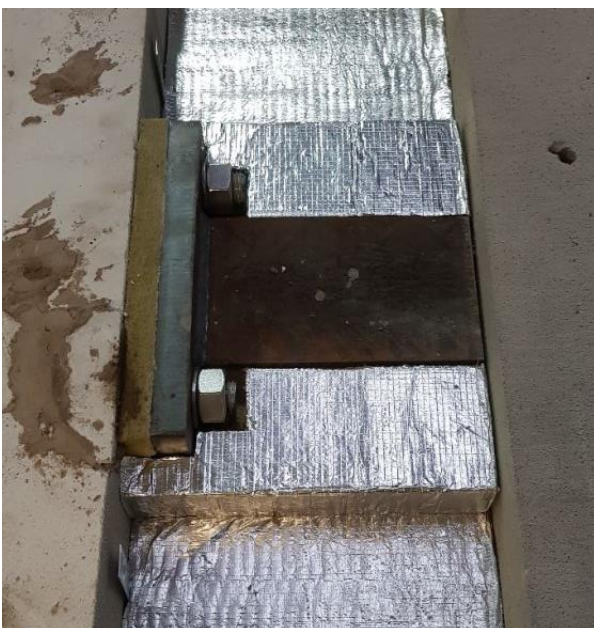
Fig 4 Stubguard® with cavity fire barrier fitted to each side
