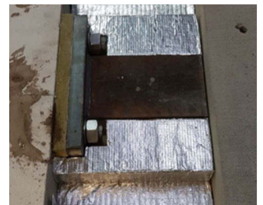
StubGuard® showing cavity barrier inserted into side face
