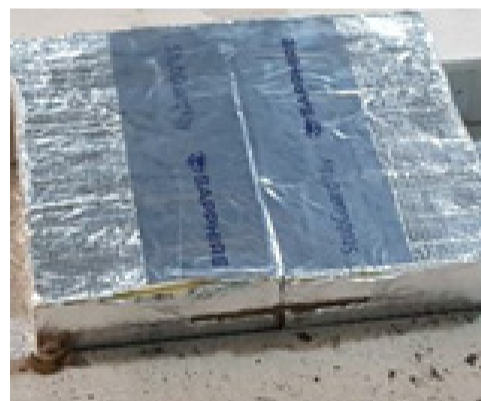
View of StubGuard® with jointing label fitted
