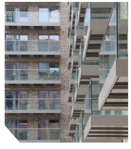
safety by containing a balcony fire and minimising its spread. The soffits help to prevent embers falling to the balcony below and block the fire from spreading to the balcony above.
