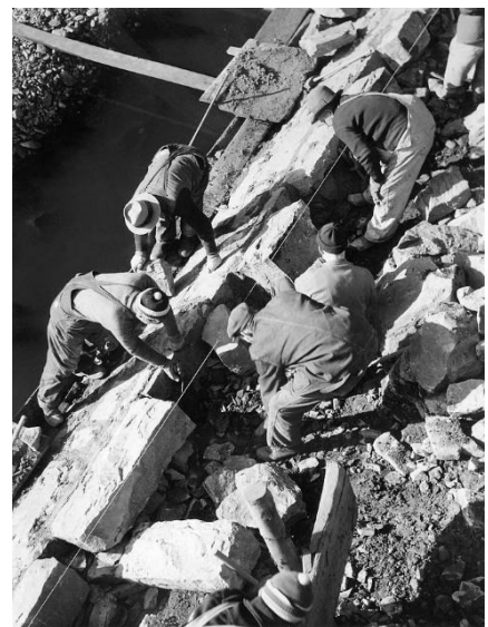
A WPA road crew at work.
