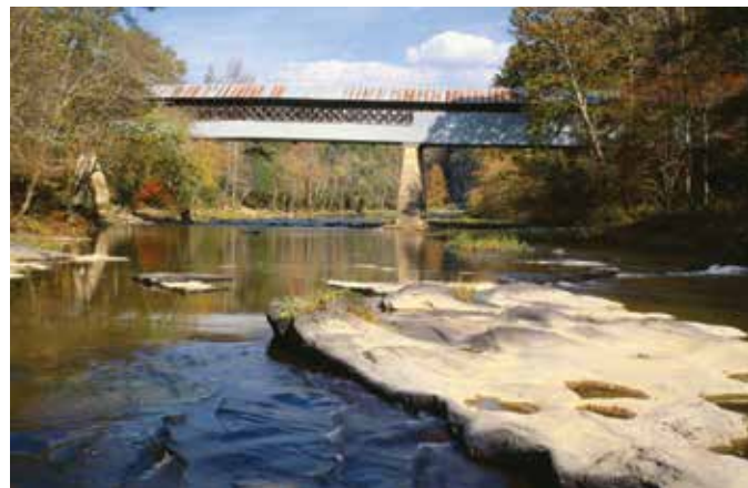
Swann Covered Bridge in Cleveland is Alabama’s oldest type structure.
