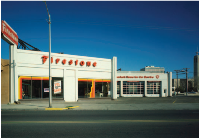
Firestone Tire Building and bell tower of the Immaculate Conception Church, 619 Copper Avenue NW (6th Street & Copper) on right, Edward J. Schulte, architect, 1957. Photograph: Copyright Carla Breeze, 2005
