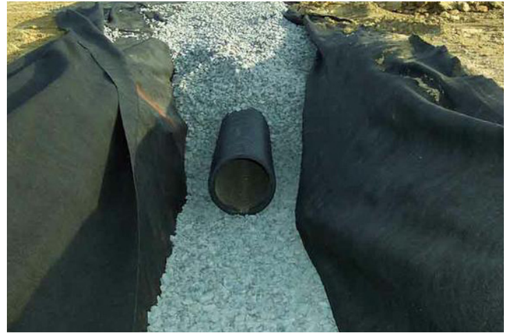
French drains are suggested in all median beautification projects.
