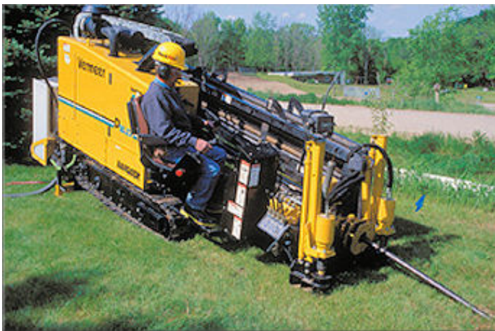
Directional drilling is the preferred method of providing irrigation and power access to areas installed without sleeves or conduit.
