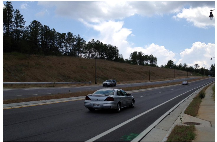
Augusta Beautification project before landscape construction.
