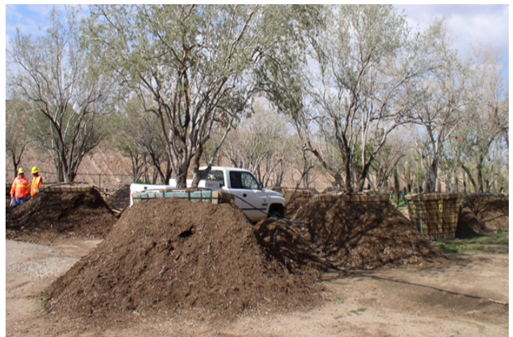
Temporary plantings or other protection are required, if plant materials are not installed within 24 hours.
