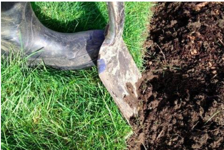
Bedlines shall be created with a three inch deep shovel cut edge.
