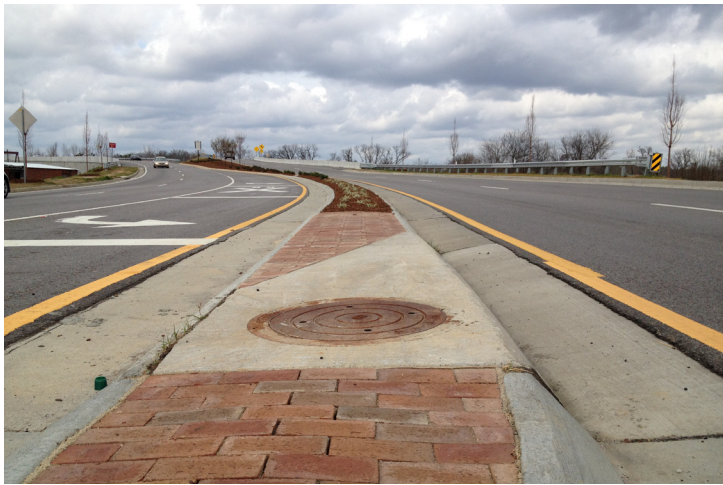
Pavers installed in a narrow median restrained by concrete curb.
