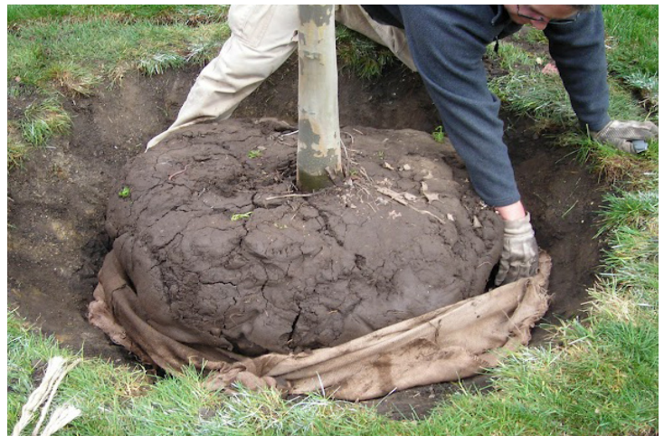
Remove the top 1/3 of burlap from the rootball during installation.
