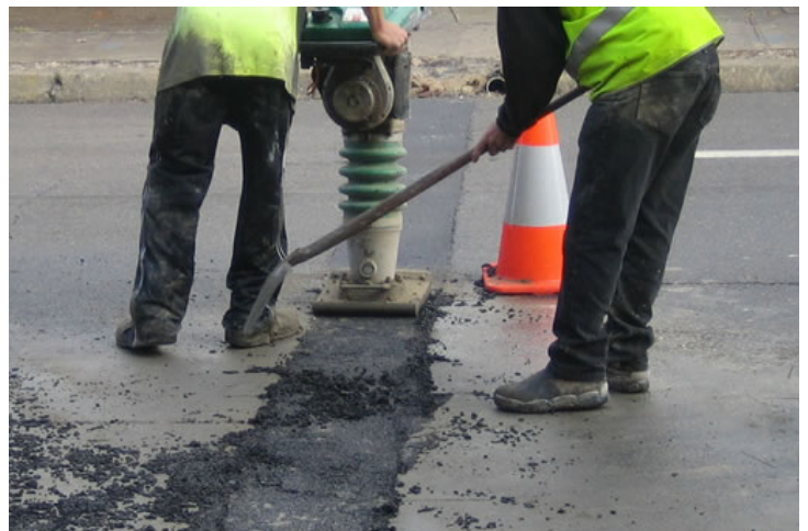
Open cuts shall be avoided at all costs through the use of sleeving and directional drilling.
