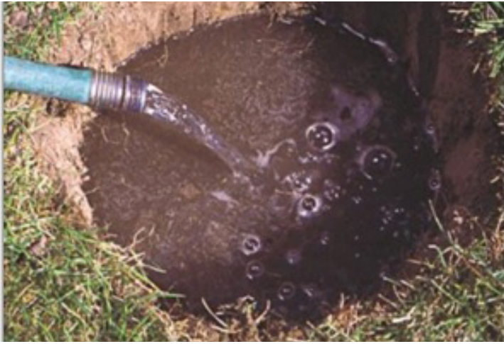
Percolation tests should be performed to determine whether supplemental drainage is required.
