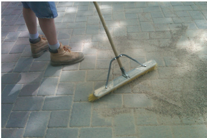
Paver joints shall be swept with polymeric sand to prevent weed growth and overall maintenance required.
