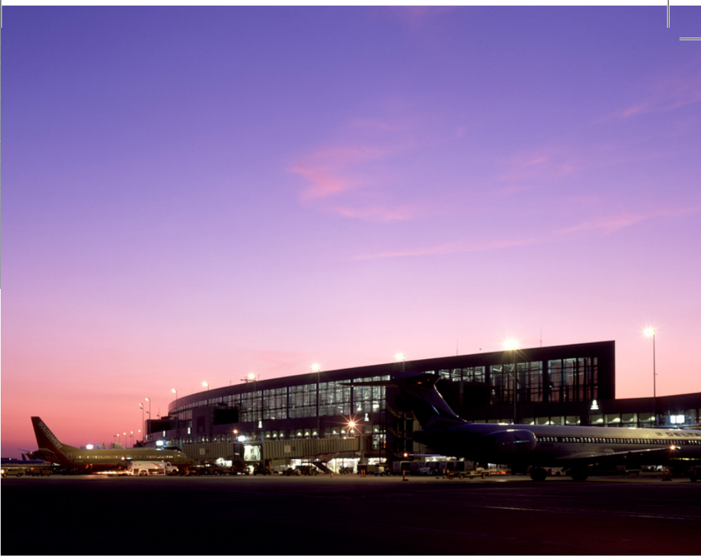
Photo by Austin Bergstrom International Airport
