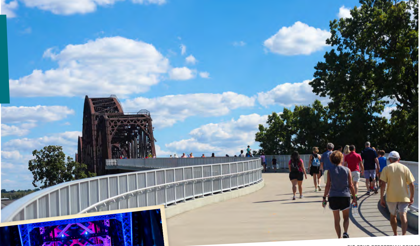
BIG FOUR PEDESTRIAN BRIDGE
