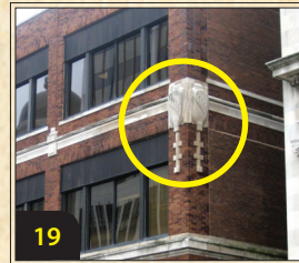
19. 113 W. Berry Street, Allen County Courthouse Annex, 1920. The fourth floor of this former Sears store was removed following a fire in 1944.
