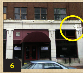
6. 118-120 Columbia Street, Flashback/Fisher Brothers Paper, 1914. Early industrial building with white terra cotta decoration.
