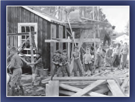
With the help of a local contractor and parent volunteers, members of Boy Scout Troop 22 built this Scout Hut in one day on May 15, 1940. They held a meeting here that night.
