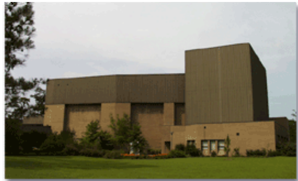
The Paul A. Johnston Auditorium at Johnston Community College – Outside View
