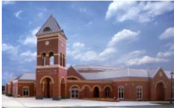
Statesville Civic Center – Outside View
