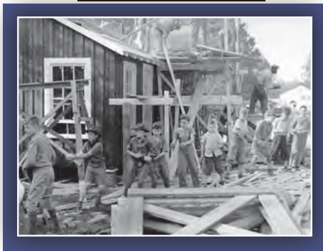
With the help of a local contractor and parent volunteers, members of Boy Scout Troop 22 built this Scout Hut in one day on May 15, 1940. They held a meeting here that night.
