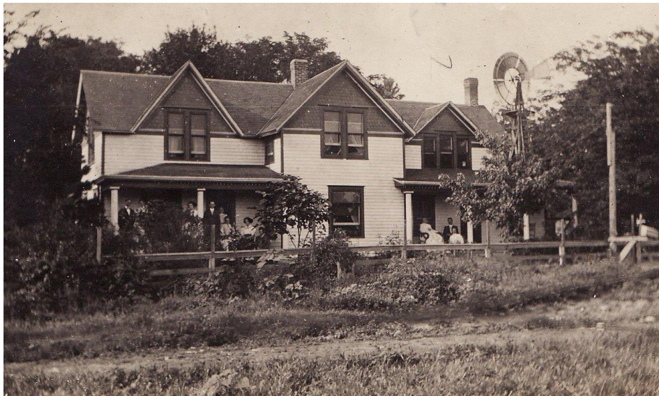
Recognized by the National Park Service's Network to Freedom Program as an authentic Underground Railroad Station
