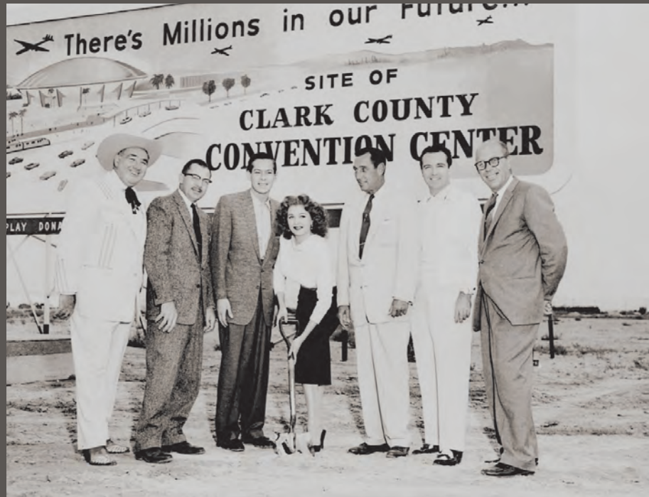
Far left: Las Vegas Convention Center / Above: Convention Center groundbreaking, 1957
