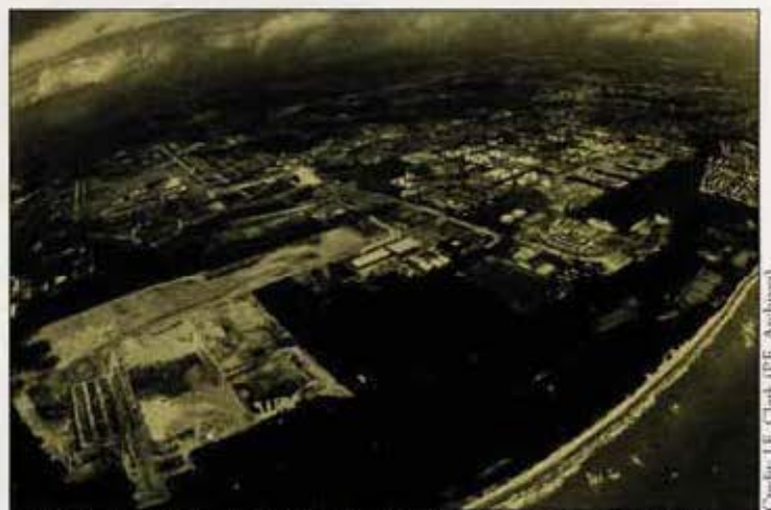
1987: High aerial shows Crowley as the pioneer tenant at Southport.
