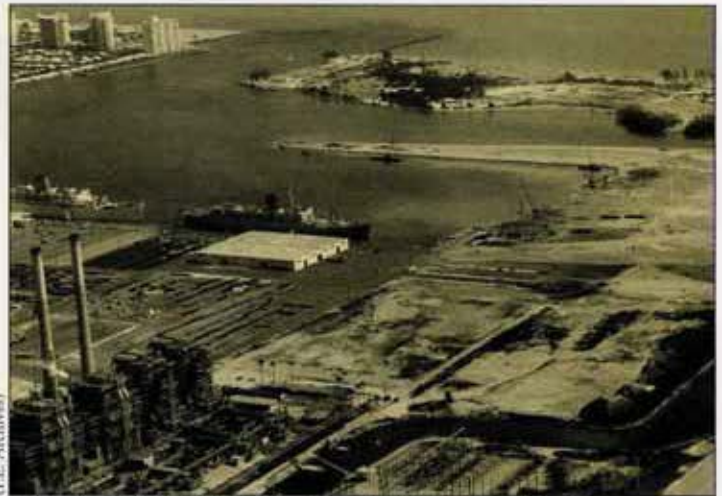
1966: A small island plot of land is removed and new Piers 5 and 7 are built in a peninsula.
