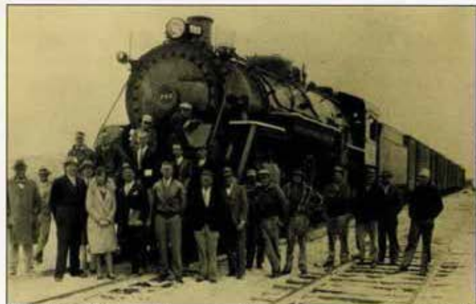
1931: On a chilly morning, port employees welcome the first trainload of cement, pulled by FEC Engine #703.
