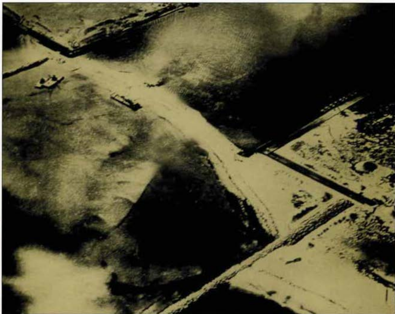
1928: The new harbor inlet is being dredged although the final barrier is still in place.
