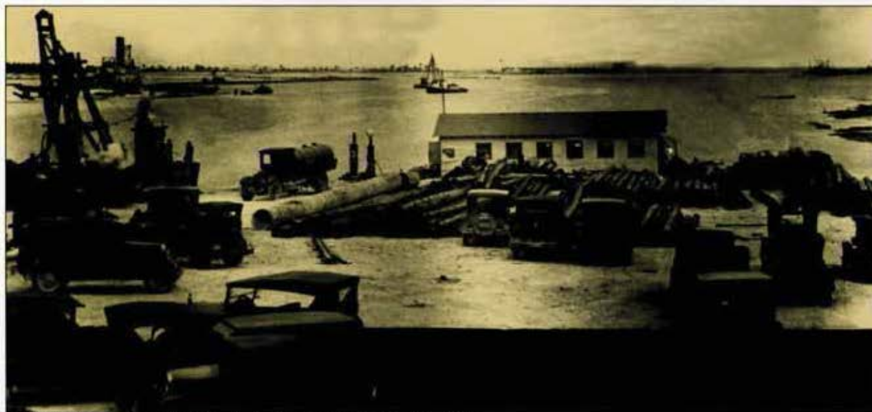
1927: Looking east from new Slip #1, harbor construction is well under way.
