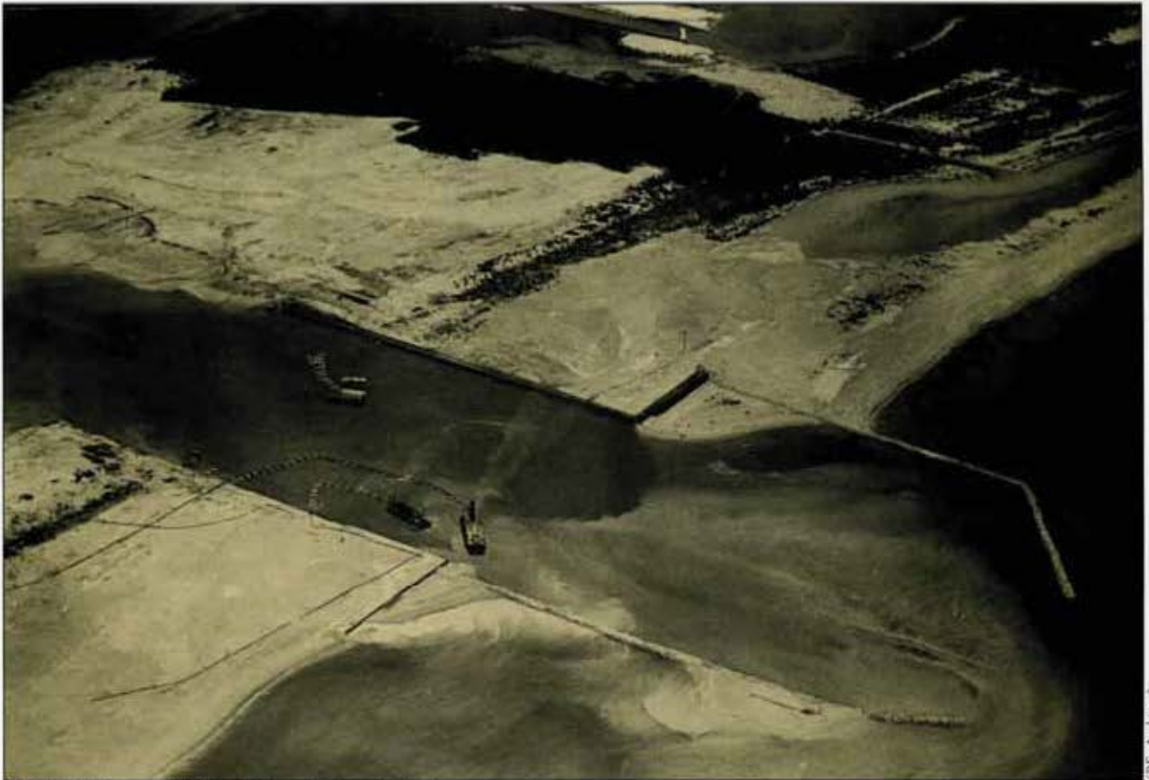
1928: Dredges steadily deepen the entrance channel.
