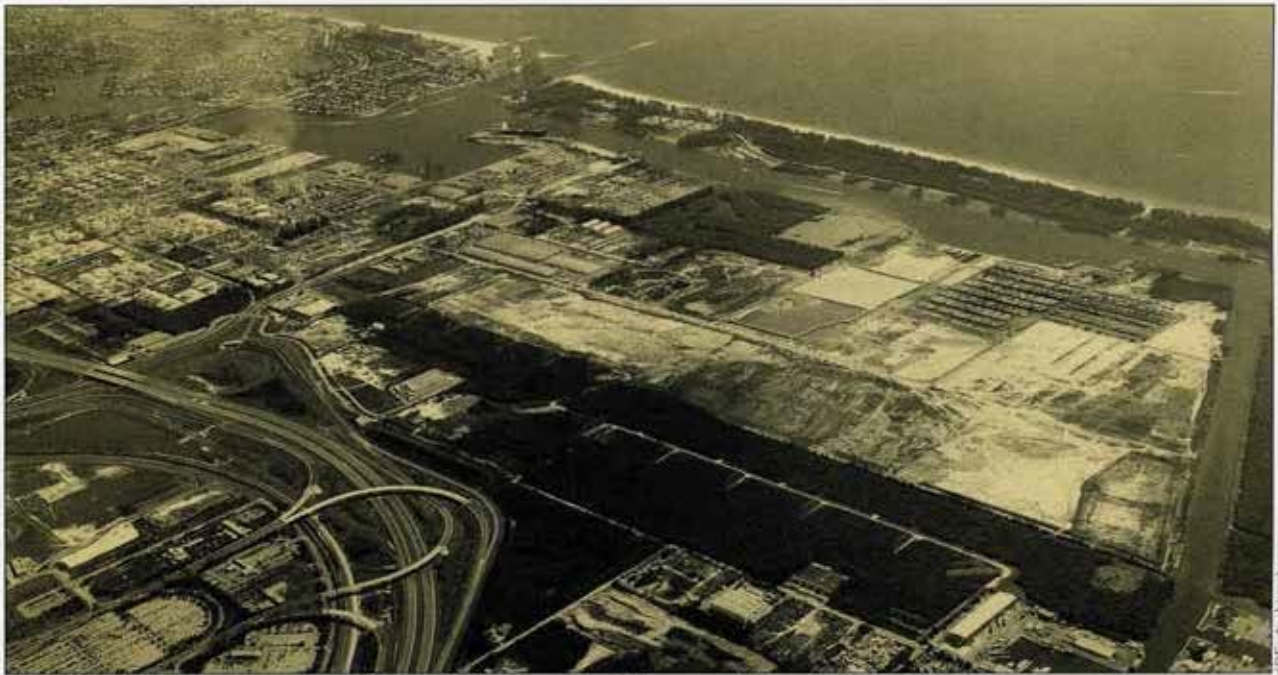
Aug. 16, 1989: Aerial shows growing 65-acre Southport terminal before new bulkhead, cranes and ro/ro ramps.
