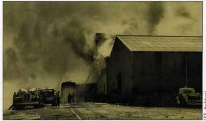
Aug. 20, 1956: Port's Fire & Security Dept. responds to a warehouse fire.
