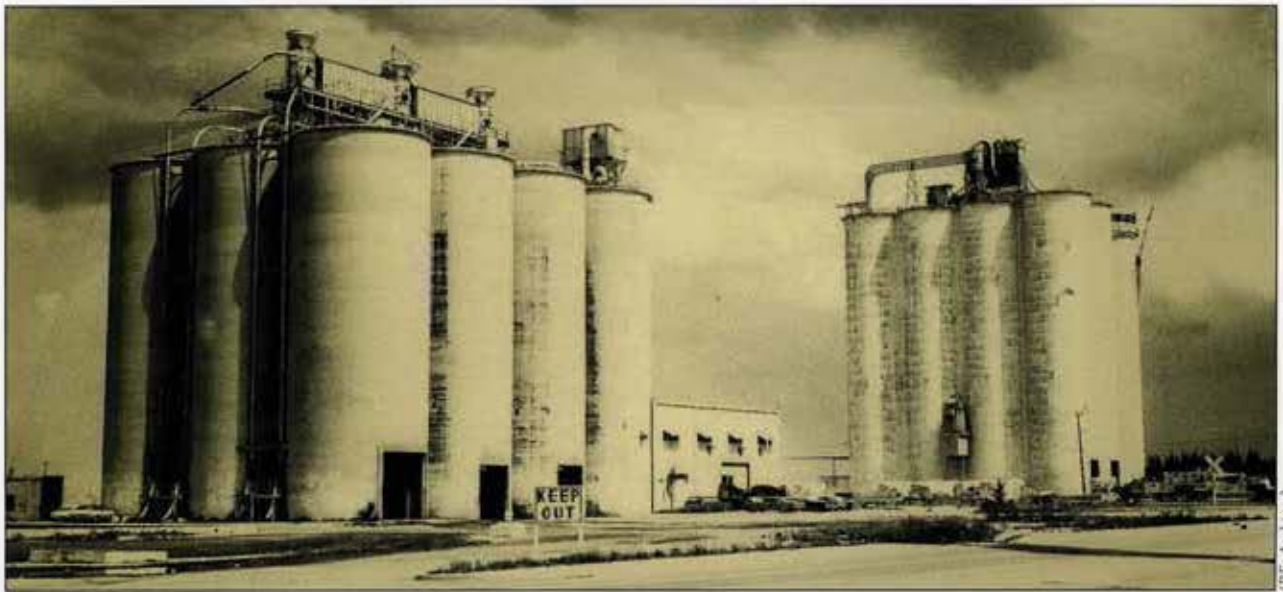
1973: Cement silos tower over the waterfront at Port Everglades.
