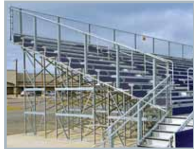
Anodized aluminum guard railing with 9-gauge galvanized chain link.
