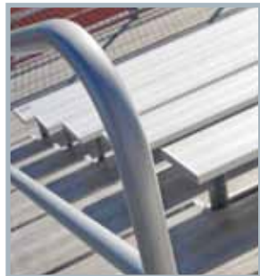
Detail of end caps on seats and mid-aisle handrail.
