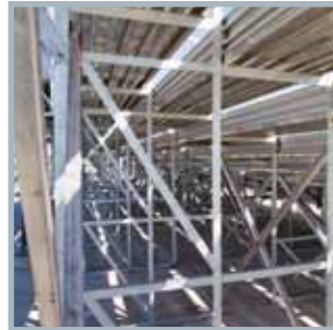
Our galvanized steel framework and aluminum cross braces.
