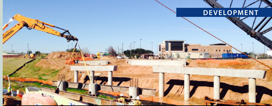
Construction on University Boulevard North
