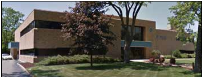
Flint - 3801 W. Boulevard - 25,000 SF 2-story office building located on 3.7 acres and includes 3 parcels north of the property for a total of 9+ acres. Wet sprinklers throughout with dry FM200 system in IT area. New roof in 2015. Diesel generator on site. Owner vacating soon. $849,000.
