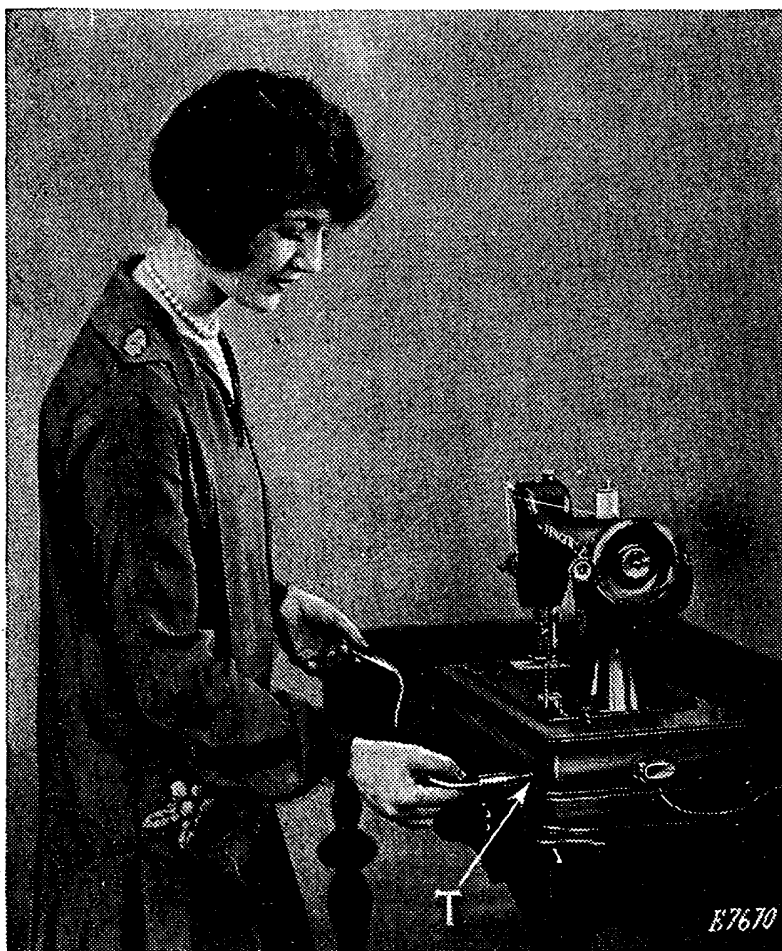
FIG. 12. PLACING KNEE LEVER IN POSITION ON PORTABLE SET 204
