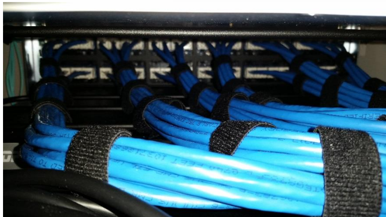
Figure 21: Copper Cables Tak-Ty to the Strain Relief Bars
