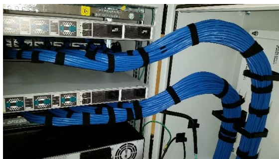
Figure 22: Switch-A (lower) and Switch-B (upper) copper cable bundles attached to the rear strain relief bars.
