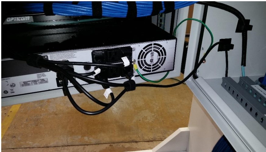
Figure 23: UPS cable routing
