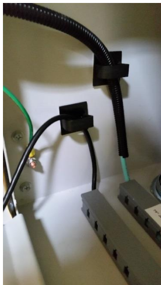
Figure 16: Fiber cable routing through the loom tubing.
