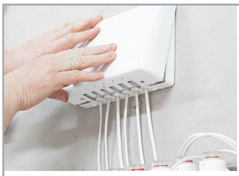
Snap on the junction box cover.
