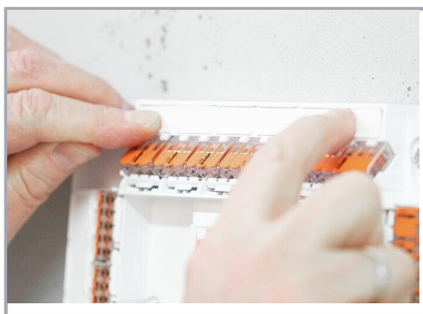
Snap the marking strips into the holder.
