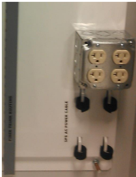
Figure 7: Outlet Box and Cover
