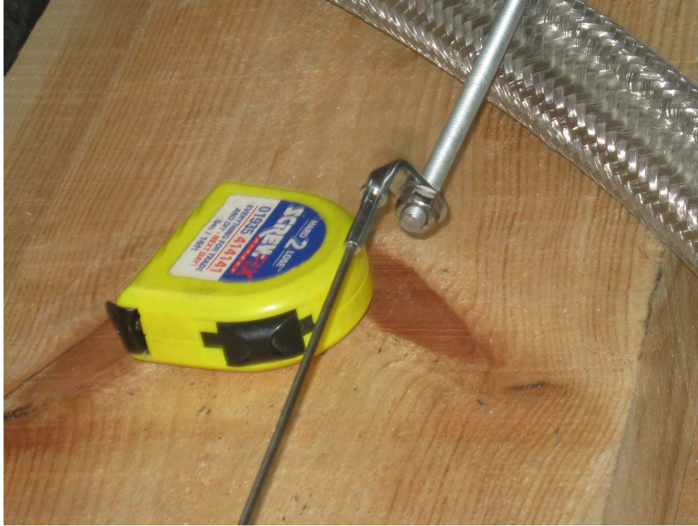
Figure 3 90° eyelet end fixing connected to M8 stud
