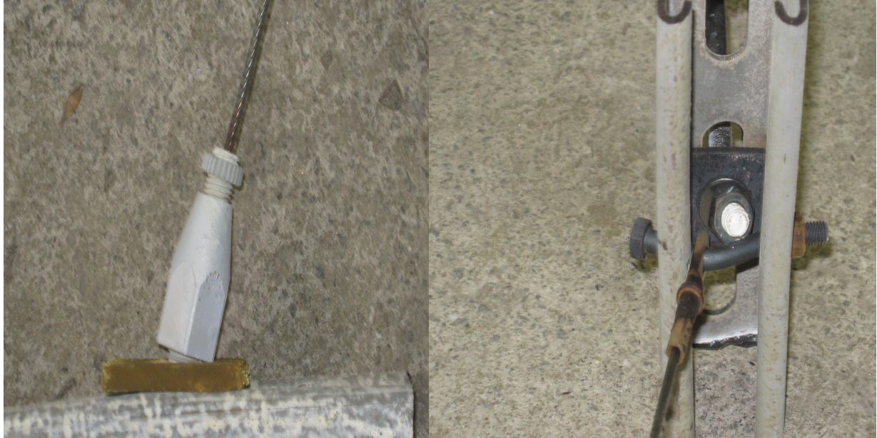
Figure 11 Fixings on removal from the furnace
