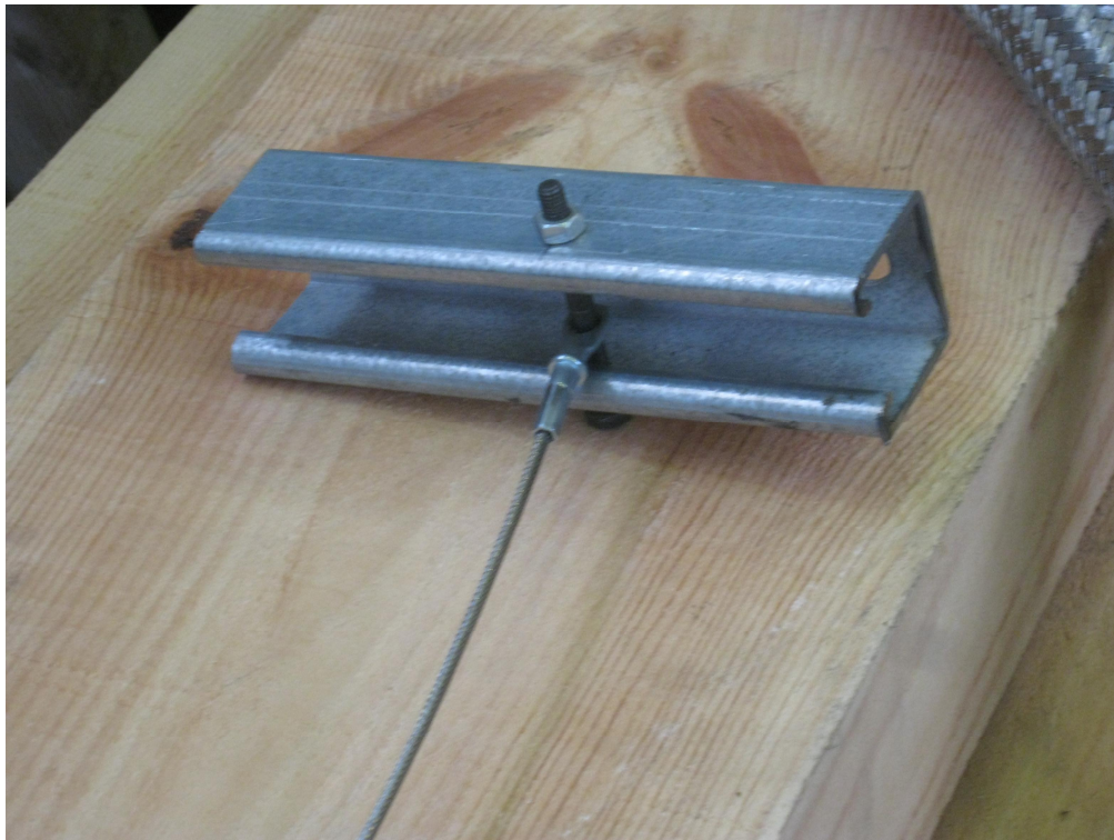
Figure 4 Straight eyelet end fixing connected to channel
