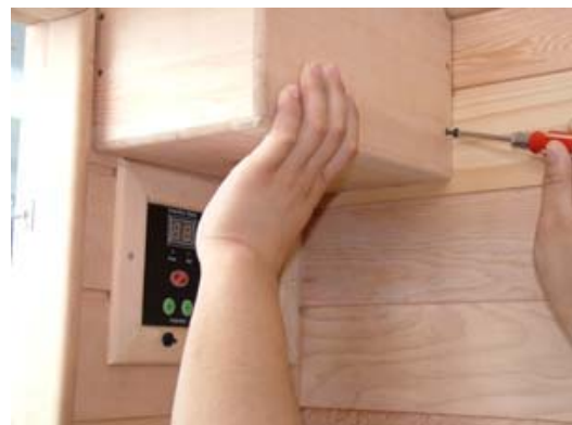
FIG-24.1 Fix the CD player back cover with screws
