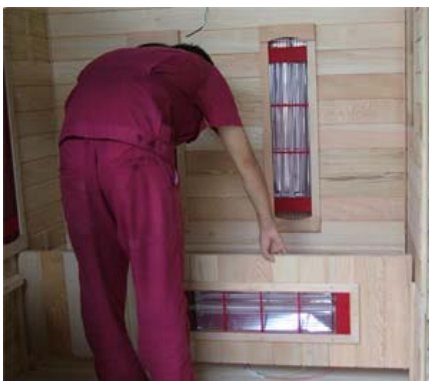
FIG-9 Assembling long sitting baffle
