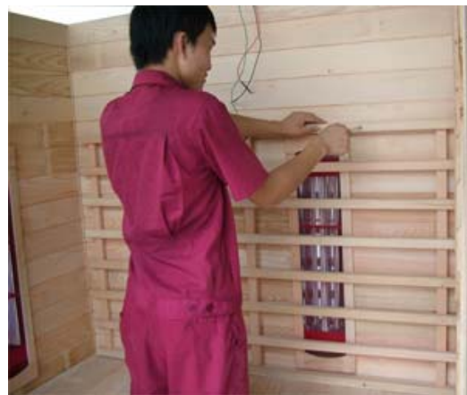
FIG-13 Fix the backrest with screws
