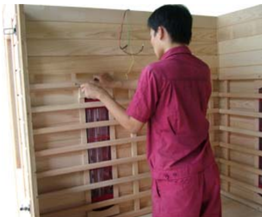
FIG-13.1 Fixing backrest with screws
