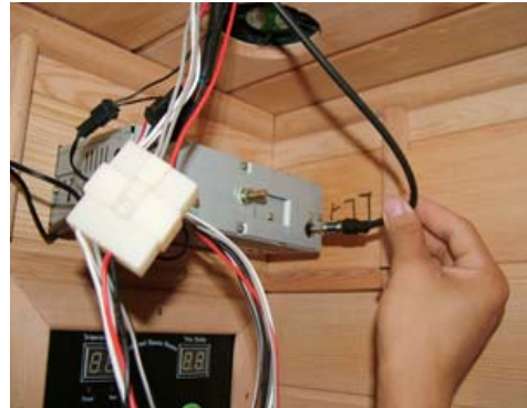
FIG-23 link the antenna connectors
