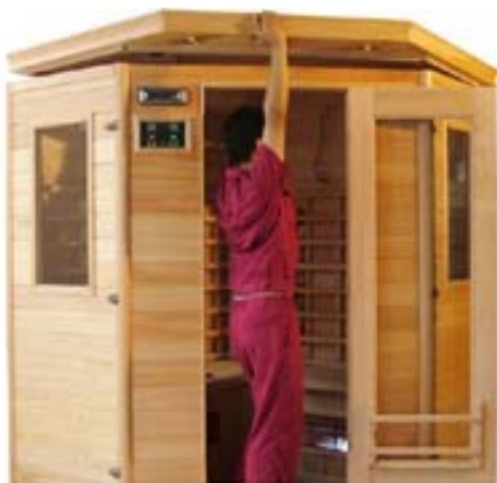
FIG-16 Assembling internal top board
