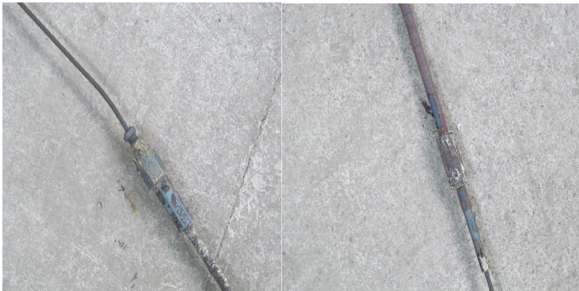
Figure 26 Gripple fixing and M10 stud fixing following 120 minutes fire exposure
