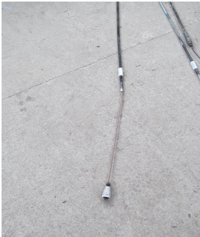
Figure 22 Gripple fixing and M10 stud end fixing following 30 minutes fire exposure
