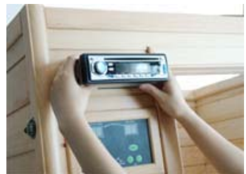
FIG-13.1 Fixing stereo w/ CD
