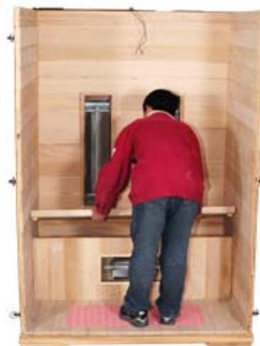
FIG-10 Assembling sitting board
