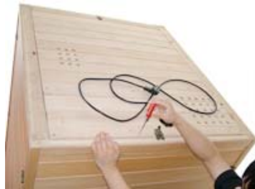
FIG-24 Fix the external board with screws
