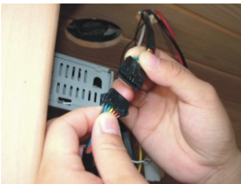
FIG-20 Link the control panel connectors
