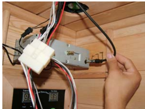
FIG-21 Link the antenna connectors
