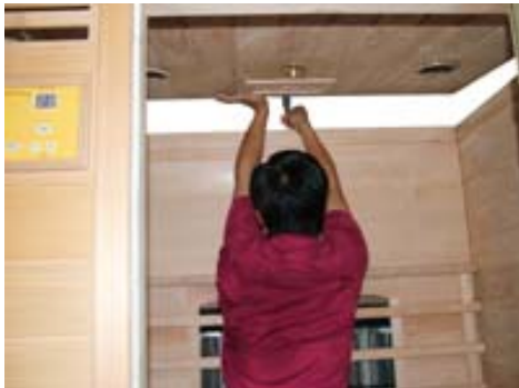
FIG-14 Setting the top board
