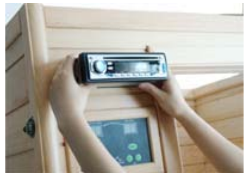
FIG-13.1 Fixing stereo w/ CD
