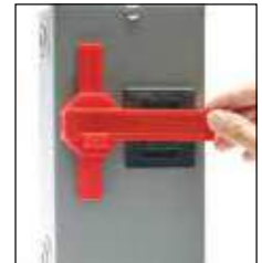
Slide Stop Bar into position over breaker
