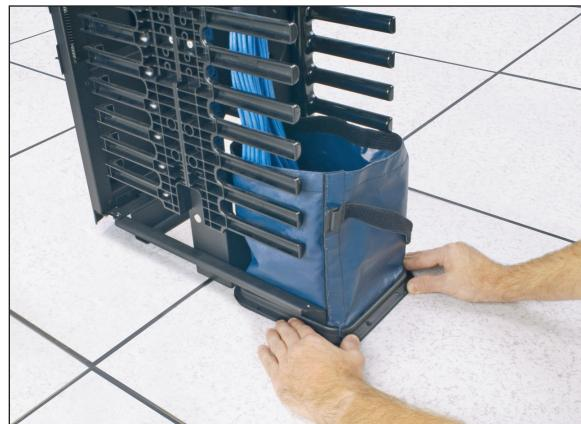
5. Secure outer ring (A) to raised floor using the self-tapping screws that are provided. This ensures a pathway to ground to prevent buildup of electrostatic charge.
