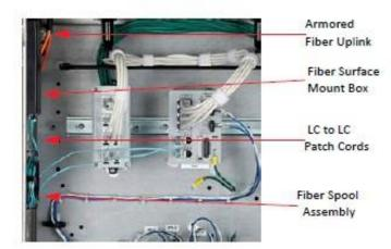
The Zone Enclosure can have either a fiber or copper uplink. Copper uplinks are limited to 330ft (100m) distance and relatively noise free environements. It is recommended to have a structured cabling approach, terminating the horizontal cable to an RJ-45 jack or LC adapter.
