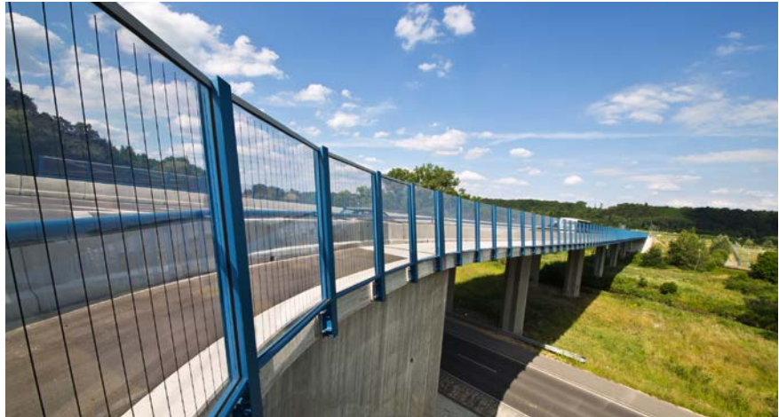
Fig. 1. Noise protection walls made of solid, transparent PC sheets withstand the effects of weather, stone chipping, and vandalism, permit a view of the surroundings, and are protected against bird strikes (© Covestro)
